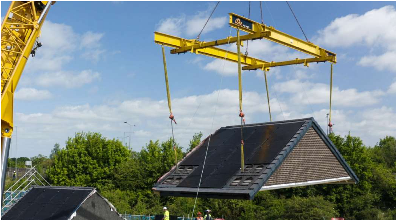
CLOCKWISE Zero-emission homes from ilke Homes are precision-engineered in a factory; ilke Homes installing a roof on a ZERO bills home, which comes equipped with solar panels
